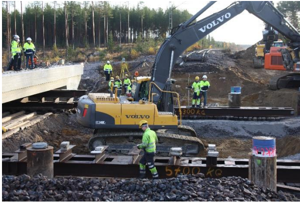
Figure 4. Kokkola-Ylivieska Dual Rail Construction – The earthworks of the bridge sites were built using BIM model-based machine automation.
